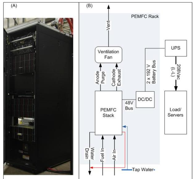
**Figure 1. (A) 10kW in-rack PEMFC system and (B) System schematic.**
